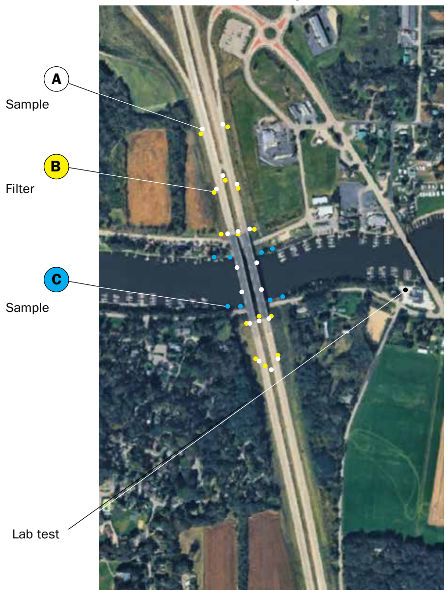
Typical Location, I-90 Overpass, Rock River, Rock County, Wi
